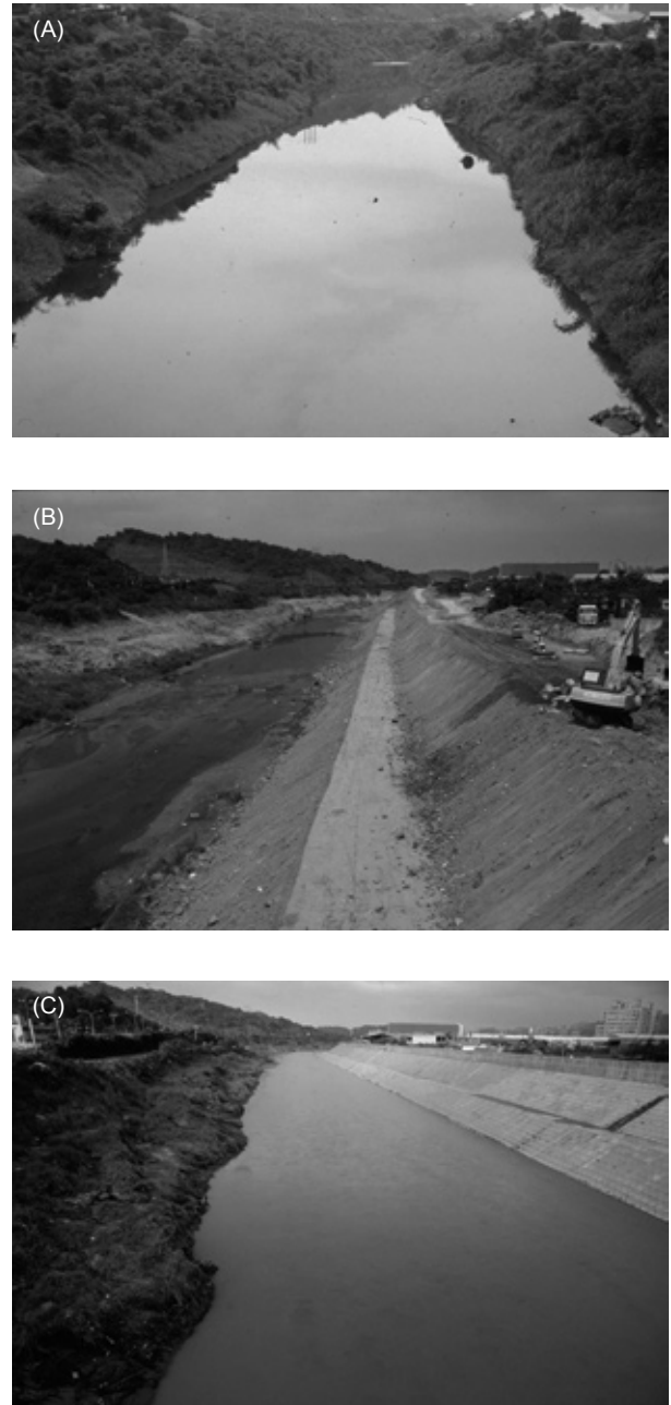
Fig. 1. Photographs of the study area (pool 1, looking upstream) showing changes in the riparian vegetation and topography of the Keelung River in (A) May 1996 (before the flood control project), (B) Aug. 1999 (during the project), and (C) Oct. 2001 (after the project).
